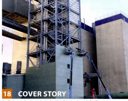
At their production site in Heijen (Netherlands), ForFarmers have built a 40-meter-high tower containing a heating line for producing poultry feed.
